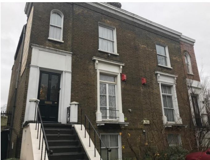
Figure 16 Nos 49 and 51 Trafalgar Avenue
