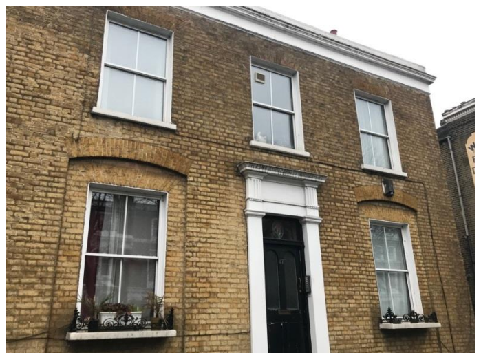
Figure 12 No. 47 Trafalgar Avenue
